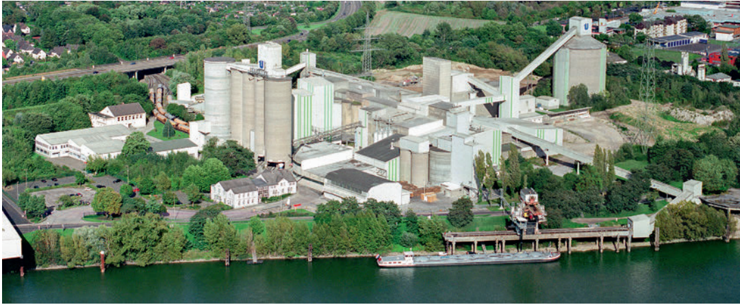
Fig. 5: Dyckerhoff cement plant in Neuwied, Germany
